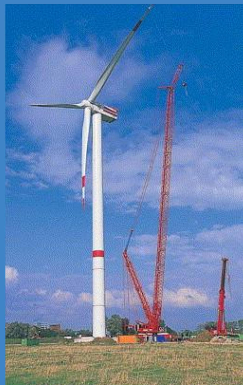
REpower's 5MW turbine with LM Glasfiber's 61.5m blade (2)
